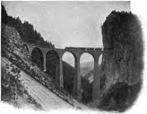
A VIADUCT ON THE NEW RAILWAY.
